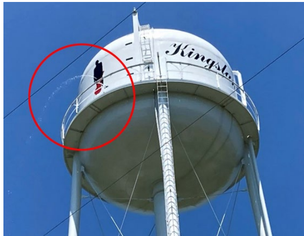
Figure 5 Leakage in water tank
